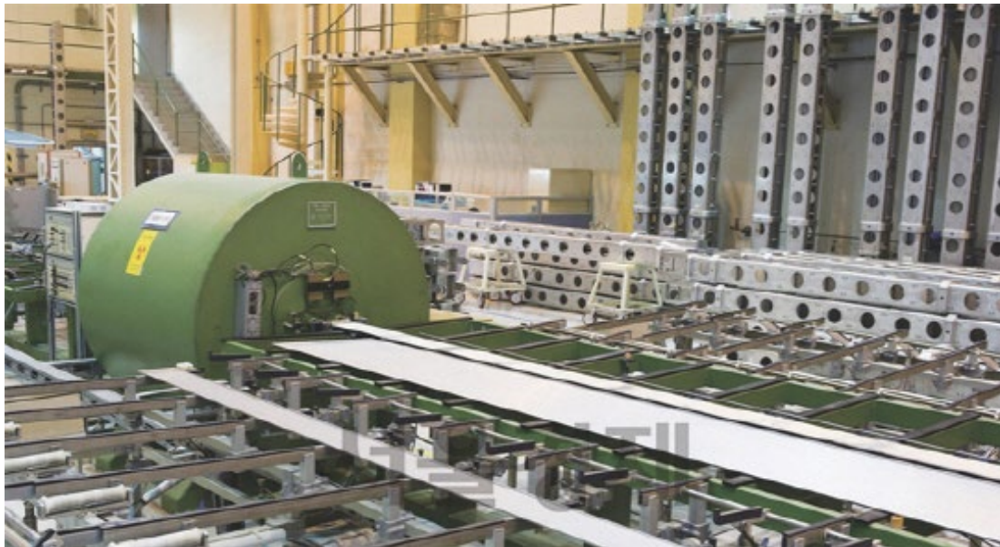
Figure 5 - Helium insertion and sealing
