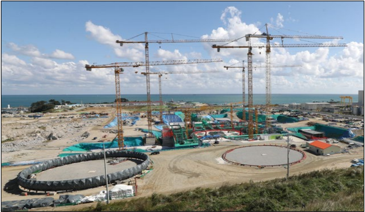
Figure 24 – Saeul 3 and 4 construction in 2018
