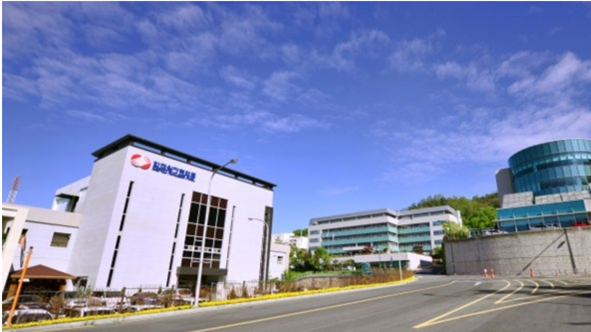
Figure 3 - KEPCO NF main building
