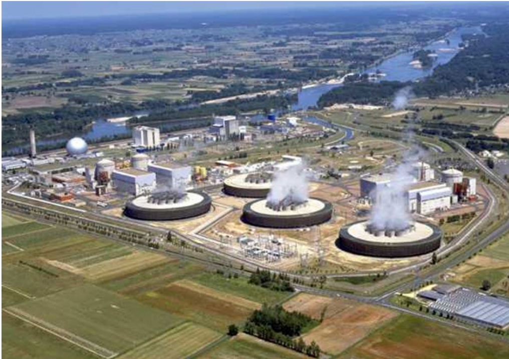
Figure 12 - Chinon B France with low profile forced draft cooling towers
